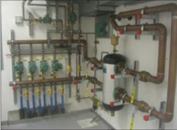
The 2-inch Caleffi Hydraulic separator provides the central organization for this elegantly constructed mechanical space. This mechanical room can be easily understood and serviced. Photo courtesy Mayo Mechanical.
